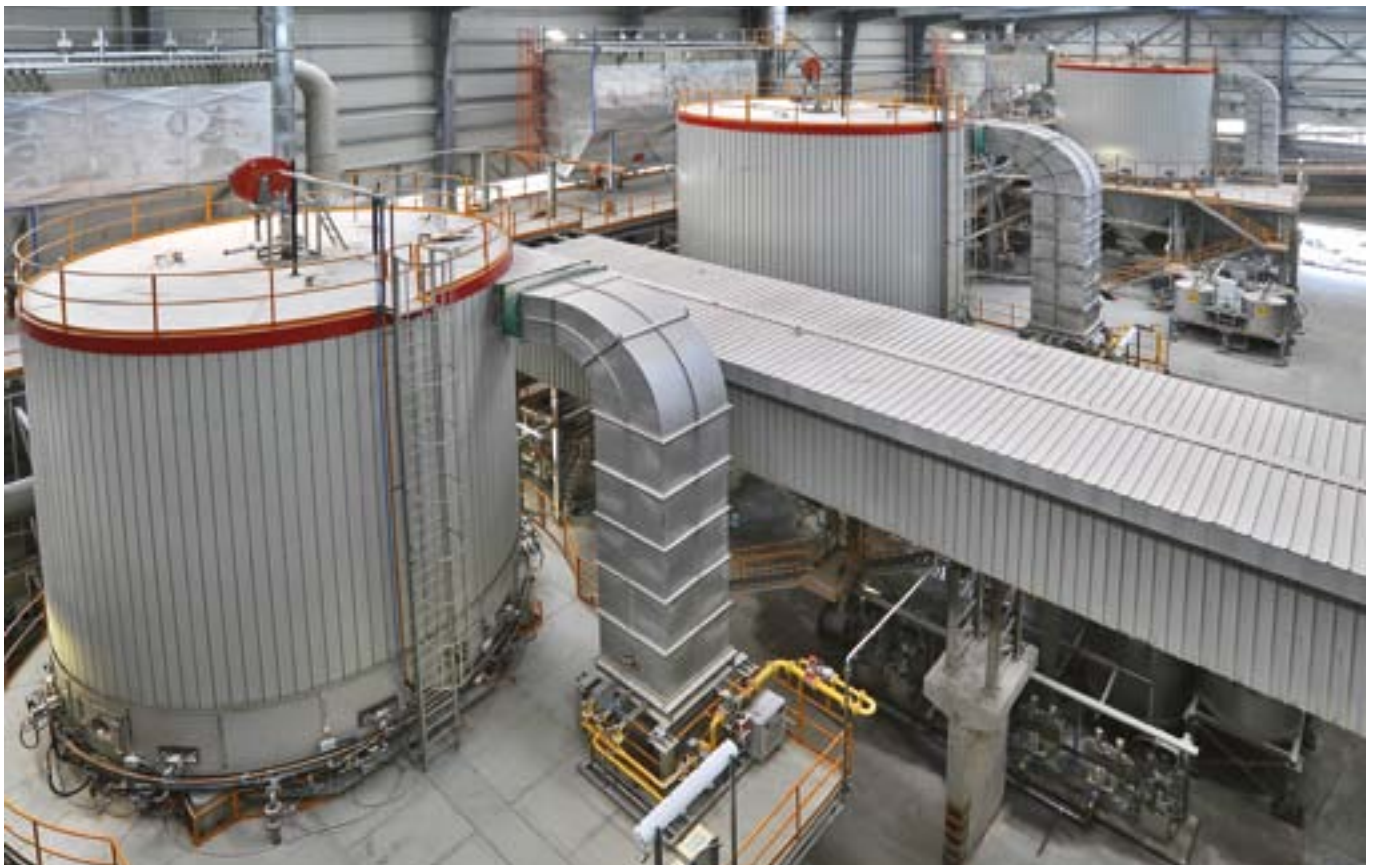
Florim Ceramiche - Via Canaletto production plant (Fiorano Modenese, MO - Italy)
